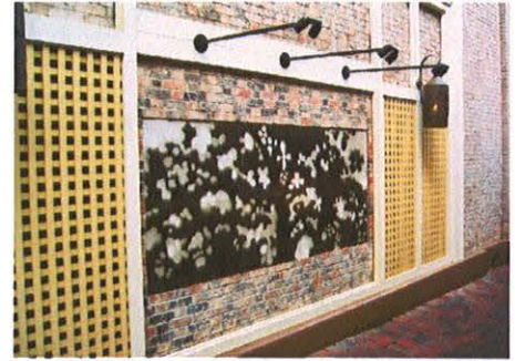
Figure 16. Wall treatment to provide interest along a walkway.
