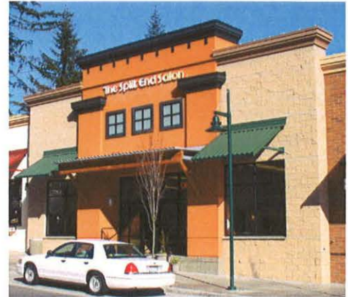
Figure 41. This storefront effectively combines EIFS and concrete block with wood trim and metal detailing.
