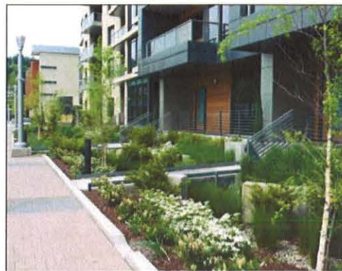
Figure 9. The preferred method of handling storm water is through retention systems, such as rain gardens, incorporated as site amenities. Other low-impact development techniques are encouraged.
