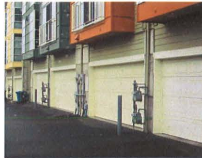
Figure 7. Place utility meters in less visible locations. Note that this example is acceptable on a service alley but not near a street or residential walkway.
