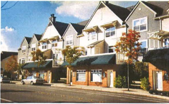
Figure 26. This mixed-use building incorporates decks, upper level setbacks, trellises, and landscaping to meet human scale guidelines.
