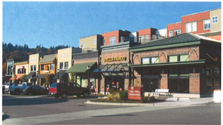
Figure 31. This Kirkland development uses a variety of roof forms and heights, different weather protection features, changing building materials and colors, and a modest amount of horizontal building modulation to reduce the overall architectural scale into smaller “storefront” components.
