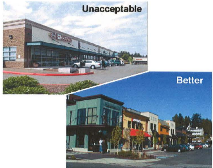
Figure 36. The continuous canopy on top is monotonous and deemphasizes individual storefronts. The bottom example provides a variety of weather protection features and represents a more desirable example.
