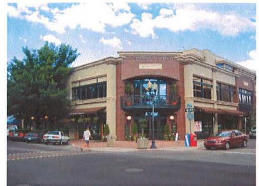
Figure 38. To emphasize its street corner location, this building uses a cropped corner, change in building materials, decorative façade elements, and a modulated roofline.
